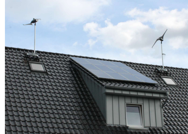
Decoupled roof-top mounted SkyWind NG turbines
