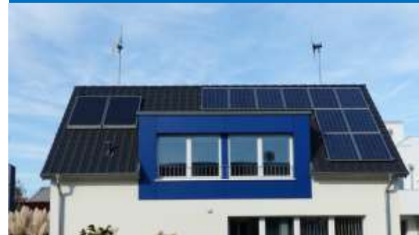
Mounted on a standard rooftop
